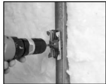
Figure 2.1: Screw clips into stud wall
