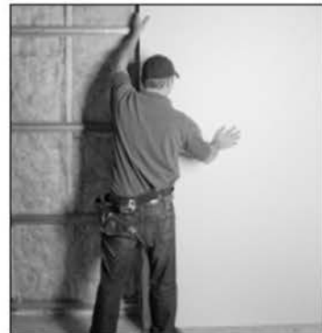
Figure 3.2: Install drywall vertically to hat channels
