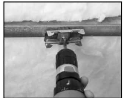
Figure 5.1: Screw A237R into joist
