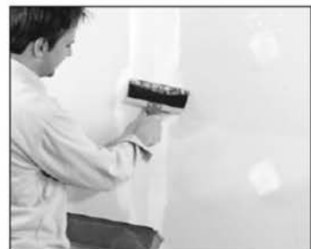
Figure 3.4: Tape and mud drywall
