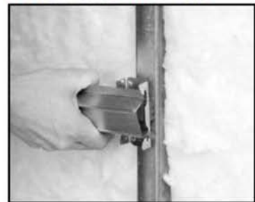
Figure 2.2: Snap hat channel into clip
